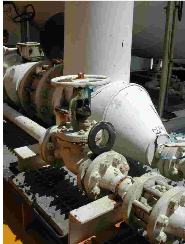
Figure 33: Spectacle blind in closed position
