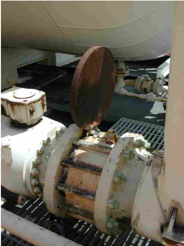
Figure 32: Spectacle blind in open position
